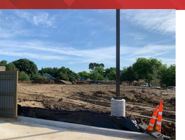
+ THE TEMPORARY **BUS LANE HAS** BEEN REMOVED AND THE CONTRACTOR IS **GRADING FOR INSTALLATION OF** THE NEW EXTERIOR BASKETBALL COURT
