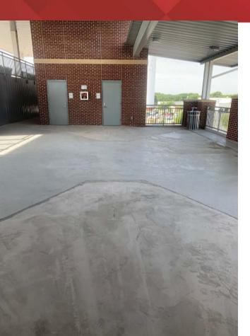
+ LANDING ON 2<sup>ND</sup> FLOOR HAS BEEN RESLOPED TO MEET ADA/TAS REQUIREMENTS. TOPPING WILL BE REAPPLIED WITHIN A WEEK OF THE AREA DRYING OUT
