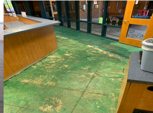
OCT flooring removal
