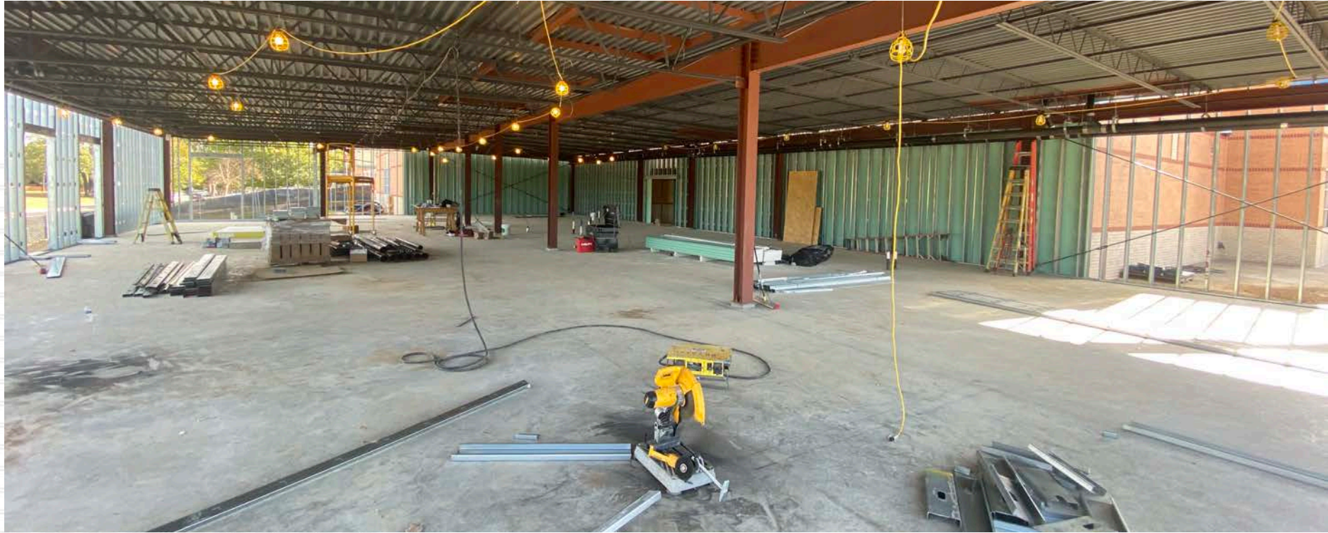
+ NEW CLASSROOM ADDITION – INTERIOR FRAMING
