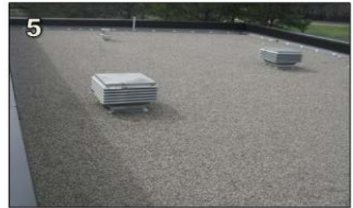
Roof top Vents.
