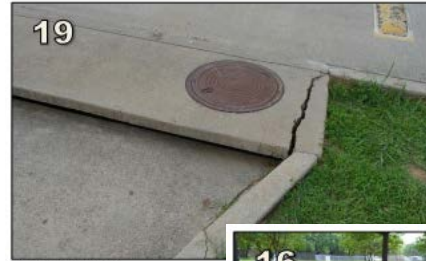
Broken curb inlet.
