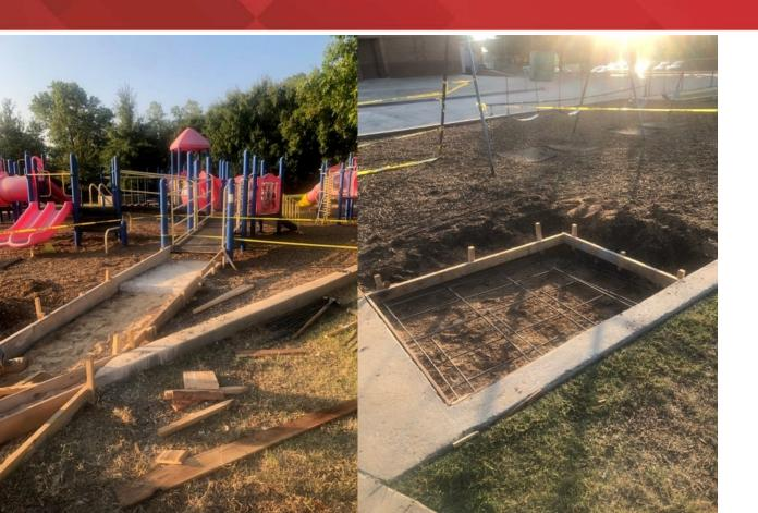
+ Accessible paths to play areas are being formed and rebar installed prior to pouring concrete
