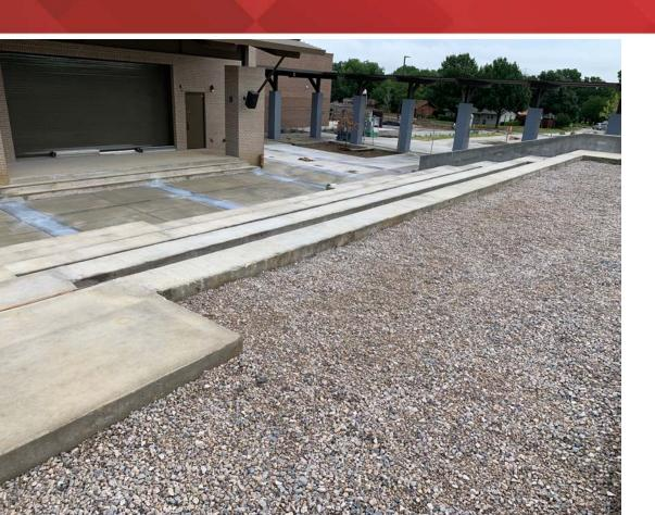
+ Top of amphitheater graded out with compacted subgrade and ready for installation of turf.
