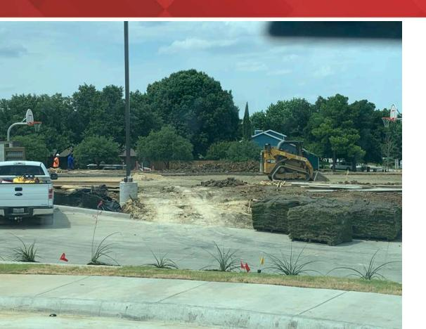
+ Grade preparation at play field to the east side of the school to prepare for installation of sod
