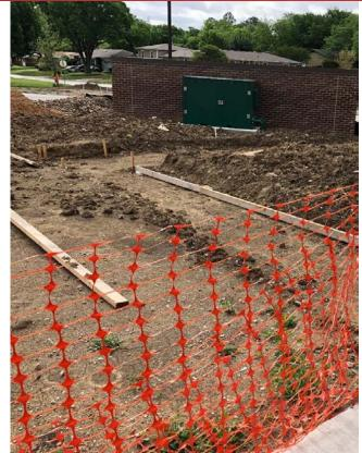
+ Preparation for a concrete paving pour on the east side canopy to the dumpster pad for access.
