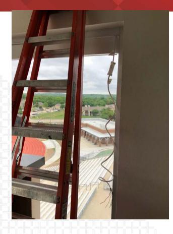
+ Power is being installed for the motorized shades at the press box.
