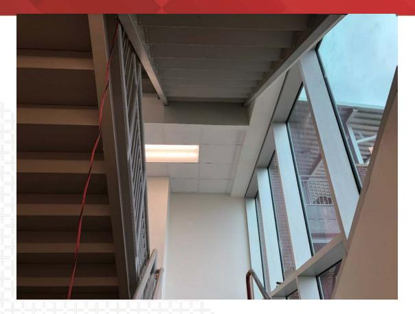
+ Exposed stairwell structure is in the process of being furred out and lay in ceiling being completed at the landings.
