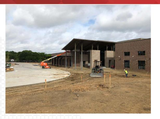
+ Front drive and parking lot complete. Front canopy is nearing completion. Front canopy on office area is complete. Grading for flatwork is underway.
